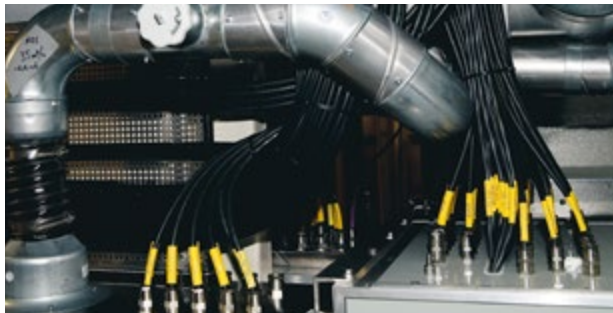
Seaguard harnesses installed
